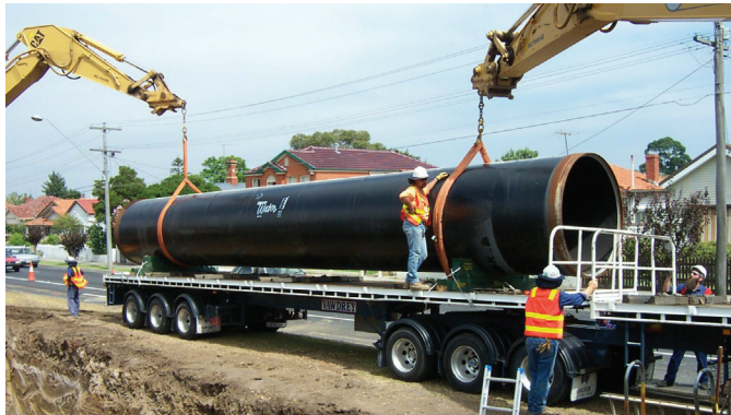
These 1700mm pipes will be used during construction.
