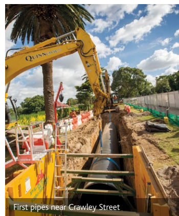
Installing pipes across High Street Reservoir
