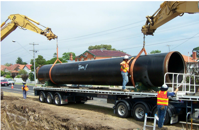
1700mm pipe being delivered
